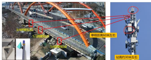
Figure 4-30 Bridge micro-deformation monitoring application case
